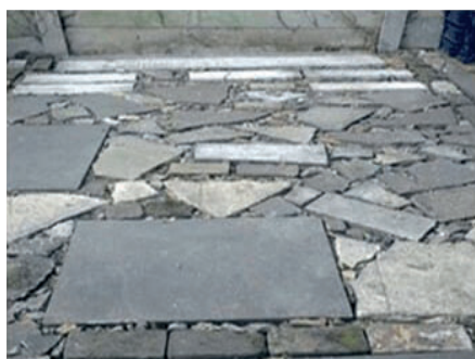
A mixture of broken slabs with no cement filled gaps
