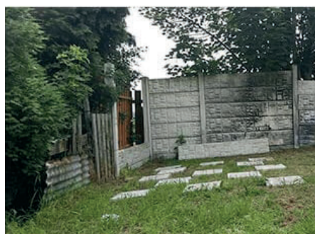
An unlevel base means the structure walls will not sit square to the floor. This will cause the structure to be unstable and pull apart over time.
