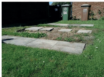
Not level due to sub soil movement beneath ground and gaps between slabs
